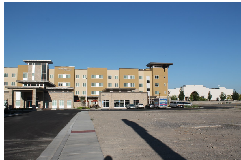
Above, Marriott Residence Inn completed Fall of 2018
